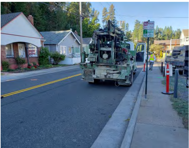
PHOTO 2.4-1: Typical Street Conditions, Looking West Along Main Street
